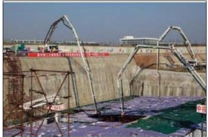
HTR-PM UNDER CONSTRUCTION
