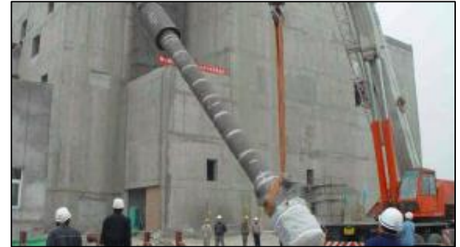
CEFR UNDER CONSTRUCTION
