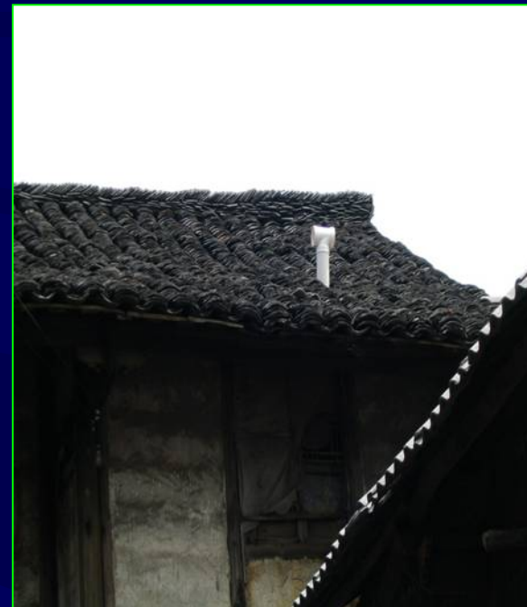
Outlet of chimney out of the room
