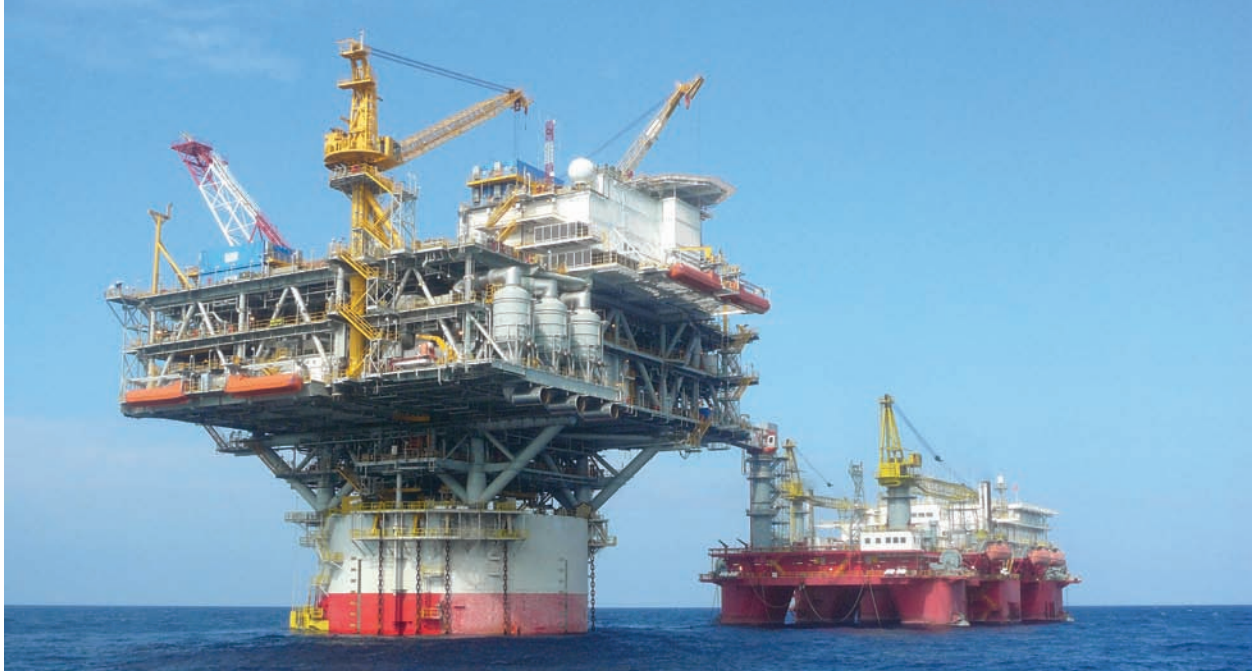
Tahiti platform in the deepwater Tahiti field in the Gulf of Mexico (2008)
