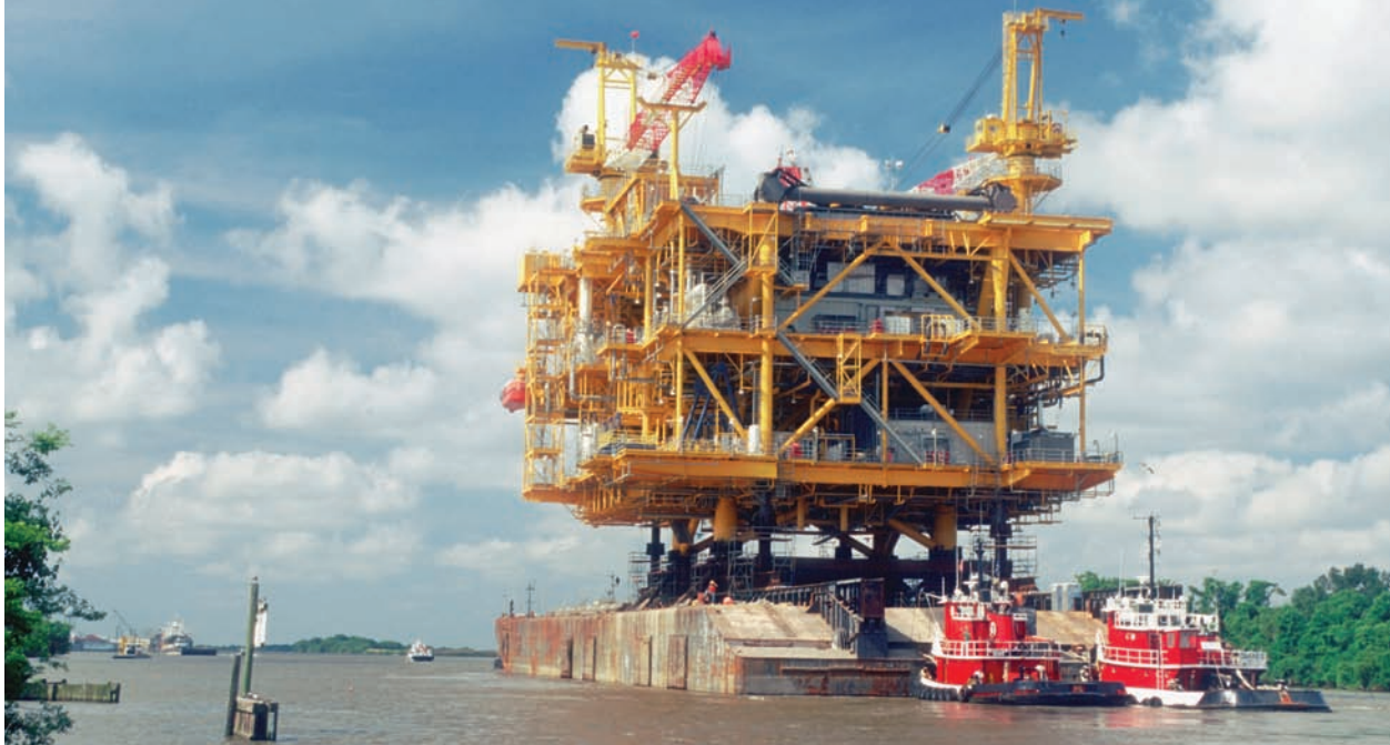
Offshore oil drilling platform being towed into the Gulf of Mexico
