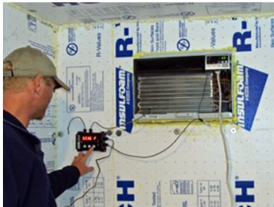
Room air conditioner controlled by CoolBot unit installed in a self-built insulated room.
