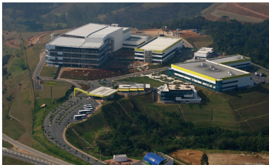
Eurofarma's new manufacturing facilities in Itapevi, São Paulo.
