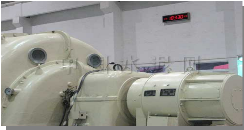
Power co-generation system
