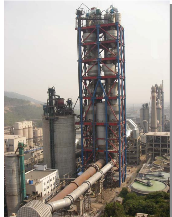
Cement manufacturing line (6000t/d)
