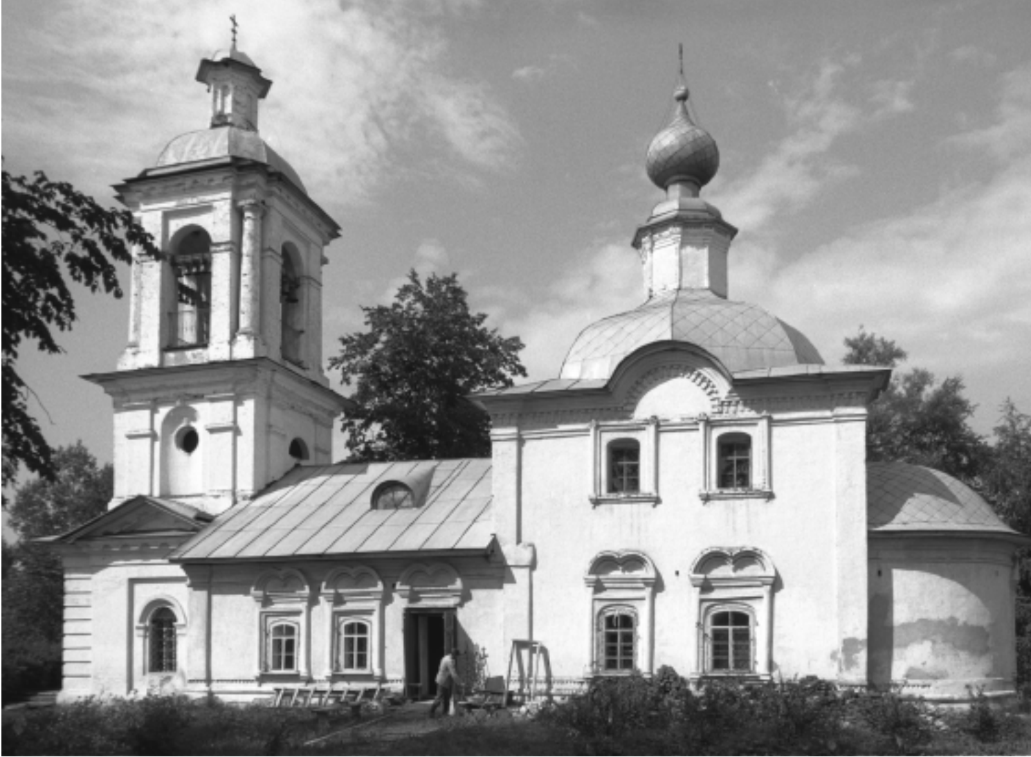
Belozersk. Church of the Epiphany. (Photo: William Brumfield)
