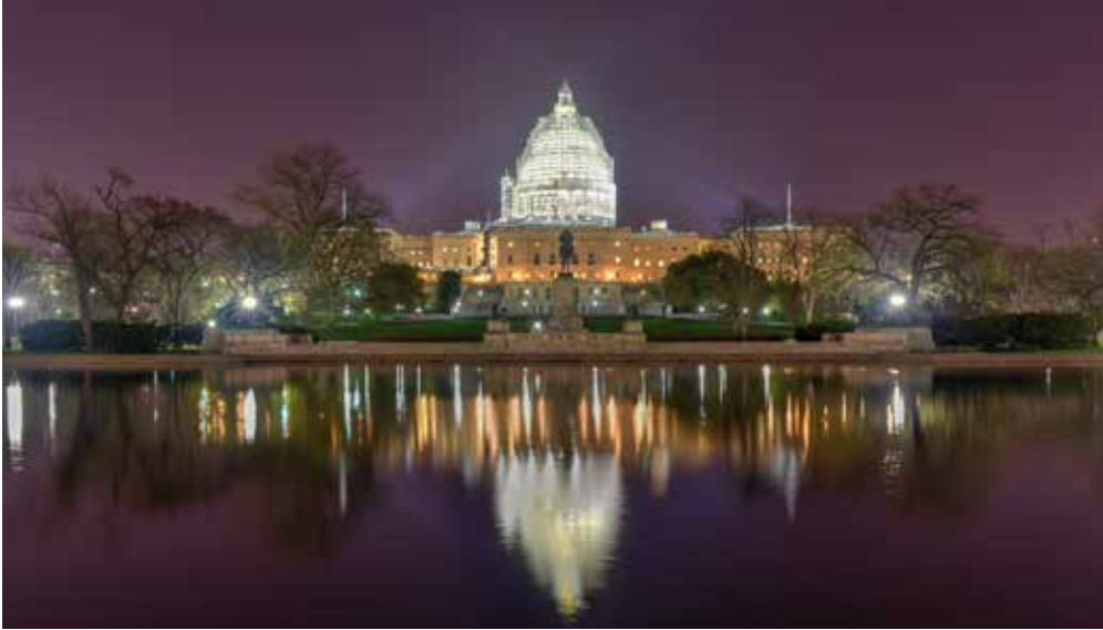
Capitol building with scaffolding, Washington D.C. Photo courtesy of Shutterstock
