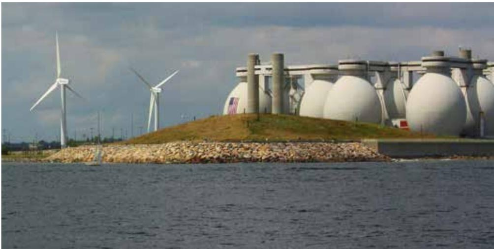
**Figure 1.** MWRA’s facilities: 98% of the plants heating needs and 22% of the plant’s electricity needs are created in-house through the process
