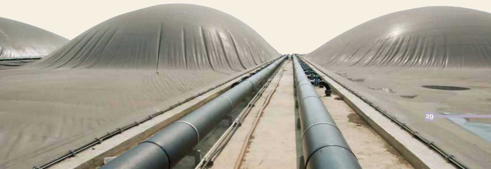
reduced water content, while the temperature of sludge is controlled below 65°C. The sludge volume is reduced significantly while the energy consumption of this process is significantly lower. Afterwards, the dried sludge can be used for composting, incineration, or building material, or as a cement additive.
