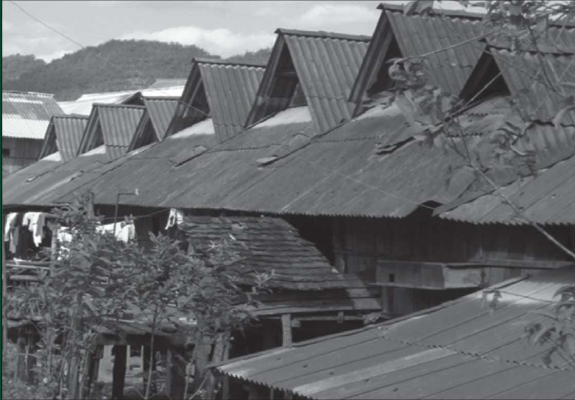
The use of asbestos as a roofing material is increasingly common in rural areas of Yunnan Province, posing health threats to both residents and the workers who produce the roofing materials. Photo Credit: YHDRA
