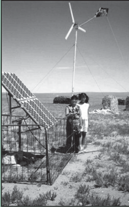
NREL has been working with Chinese counterparts to promote rural electrification, such as this wind and solar initiative in Inner Mongolia. Photo Credit: NREL
