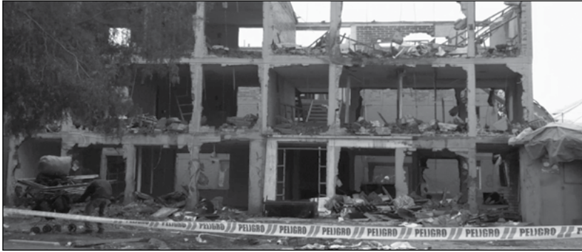
Figure 6. Social Housing being demolished in Bajos de Mena, Santiago de Chile, during 2013
